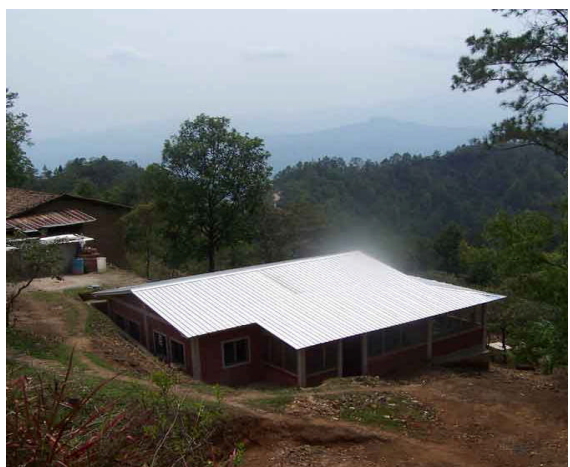
Volunteer house nearing completion
