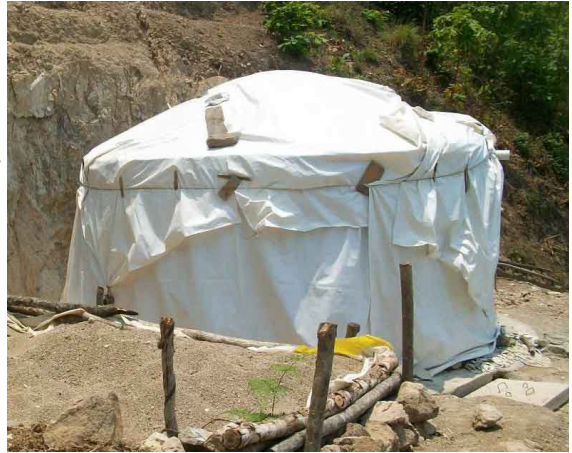
Guanacaste water tank wrapped in plastic to cure
