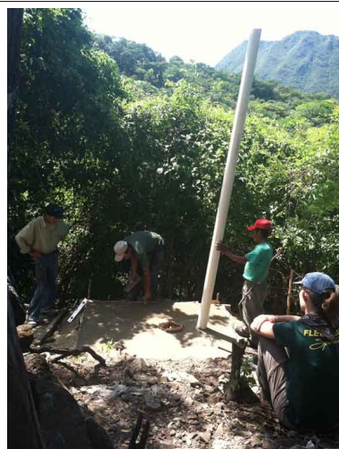
Latrine being built in Delicias
