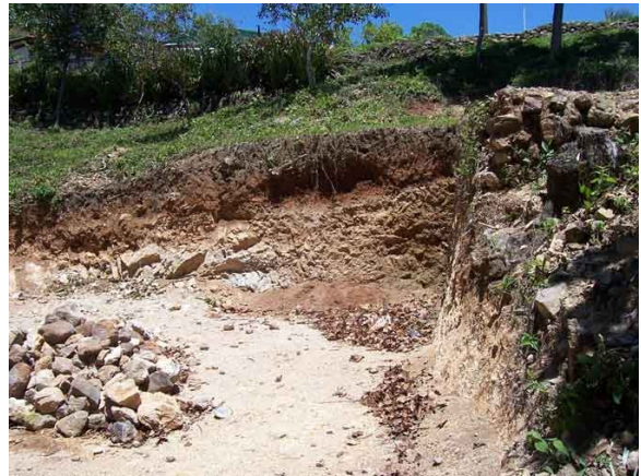
10 ft deep excavation for volunteer house
