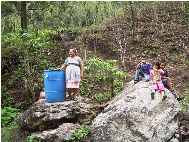
Slow sand filter in San Jose Centro
