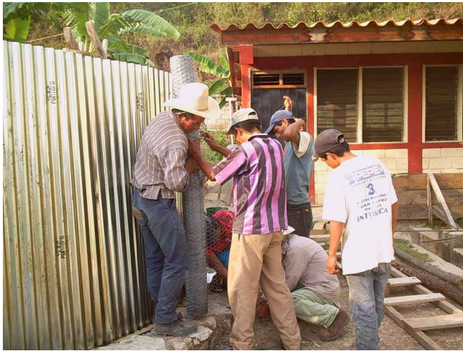
Wrapping chicken wire around the form before plastering
