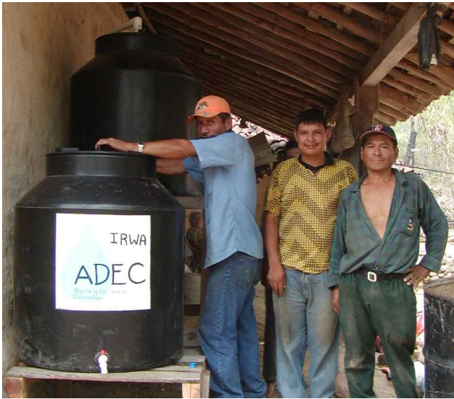
Flocculation & chlorination tanks ready for use
