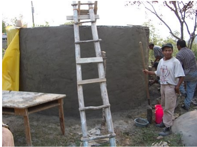
Ferro-cement tank being plastered
