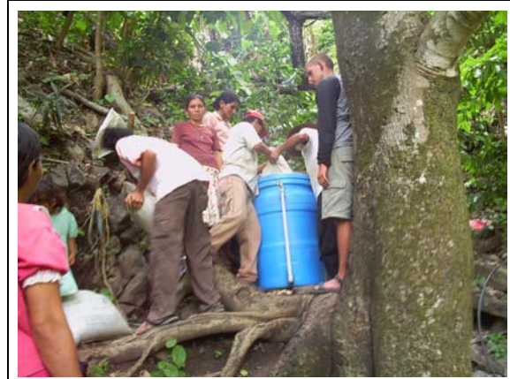
Building a slow sand filter at the water source
