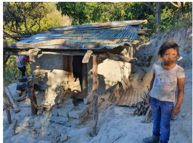
Potential future solar system install site
