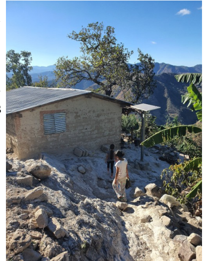
Solar system installed 5 years ago by another group at an isolated home
