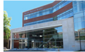
CTSI is housed in the Saunders Research Building.
