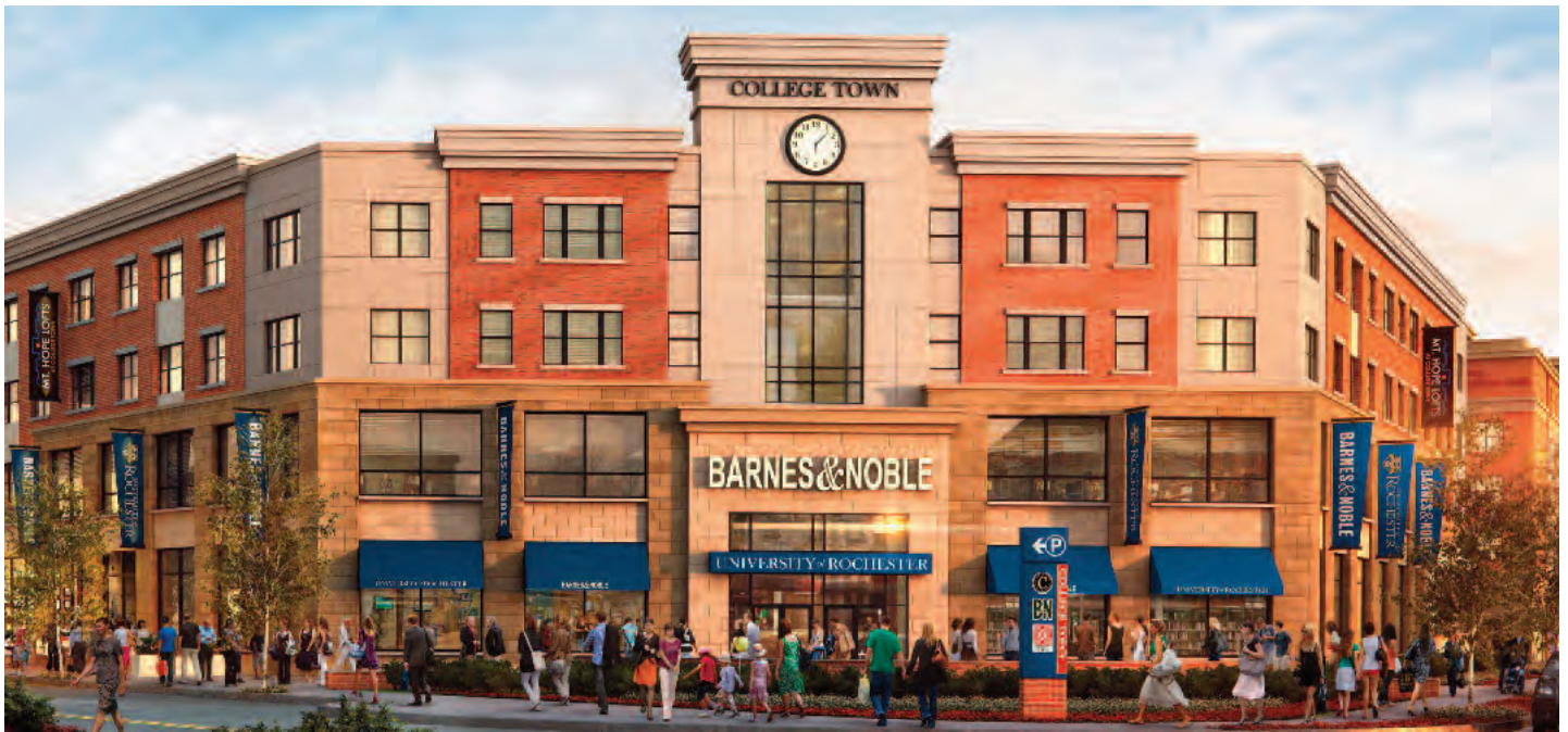
Below: A panoramic view shows the extent of the College Town construction.
