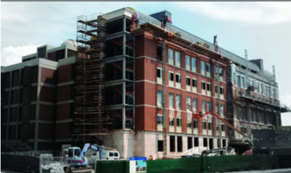
Construction on the Robert B. Goergen Biomedical Engineering and Optics Building.
