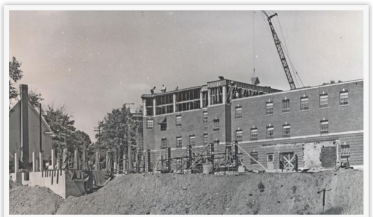
Addition of the third floor
