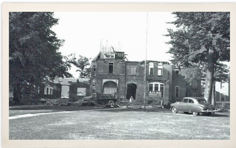
Original hospital buildings under demolition
